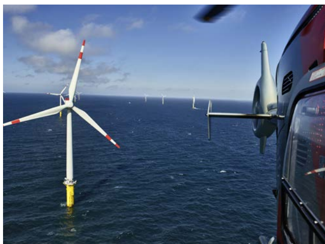
Offshore-Windpark Borkum West in der Nordsee | Foto: © Adwen/Jan Oelker
